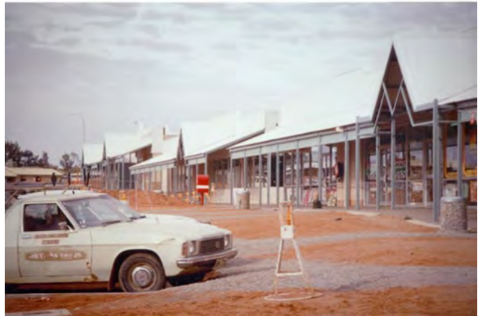
Richardson Place Construction circa 1987/1988 (source Travis Hague)
