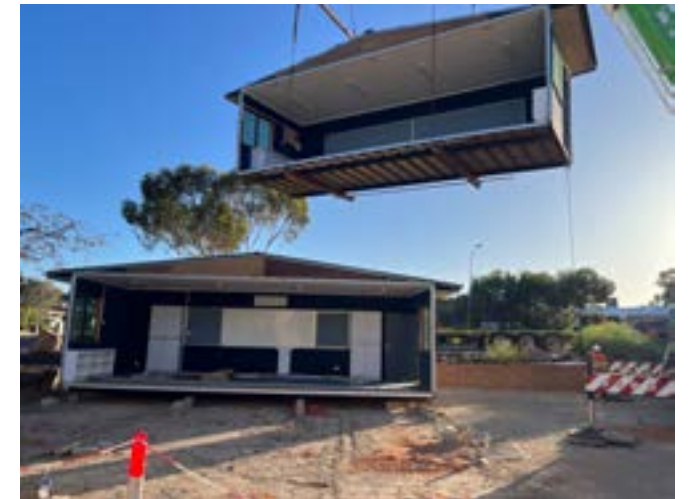
Image above: Transportable buildings being installed at Roxby Downs.
