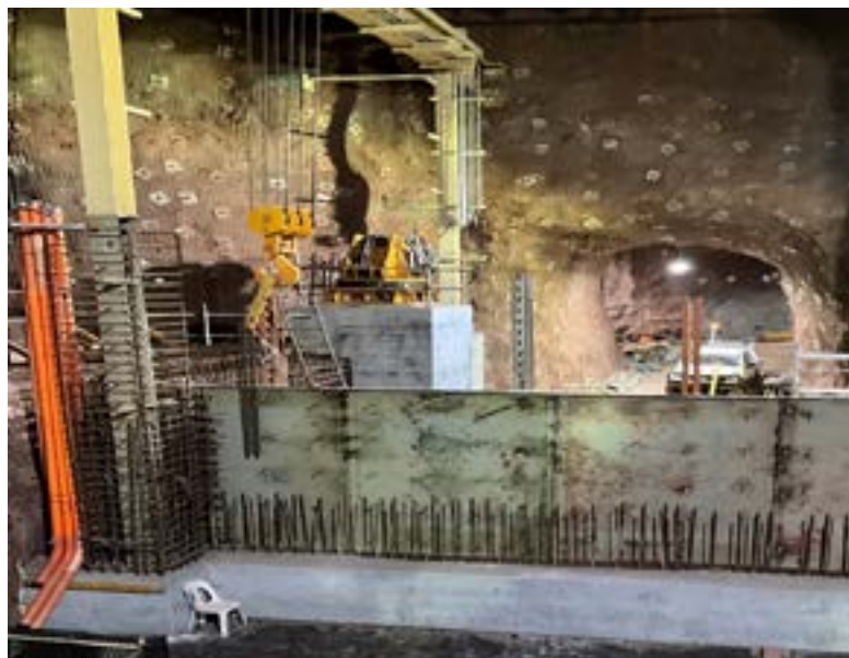
Image above: The Crusher "Dump Pocket" wall 4195-CCH-200.
